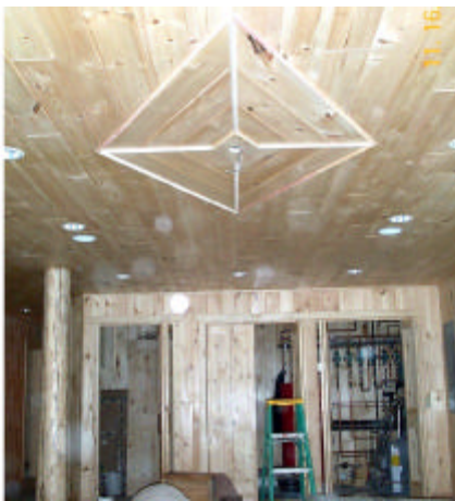
Diamond in ceiling of family room
